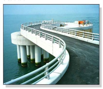
Tohoku Electric Power Co.,Ltd Location: Fukushima Prefecture Dimensions: Total length 44.754m Total width 4.0m Girder length 25.8m (Post-tensioning) Girder length 12.9m (Pre-tensioning) Materials: CFCC  $1 \times 7 \phi 12.5 L=7,596m$ CFCC 1 × 7 φ12.5 L=1,625m Application: Post-tension(main gilder) Pre-tension(main gilder) Completed: Dec 96 ACC Projects list:
