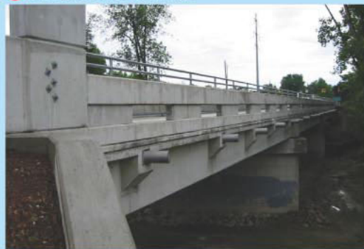
① Bridge Street Bridge
